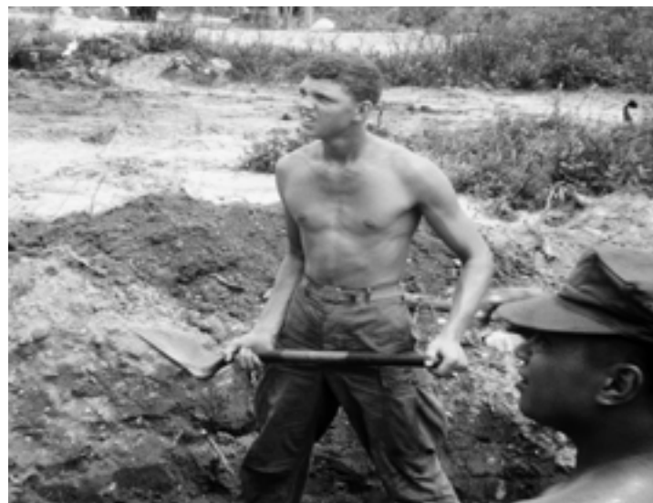
Rick Lewis in the trenches
